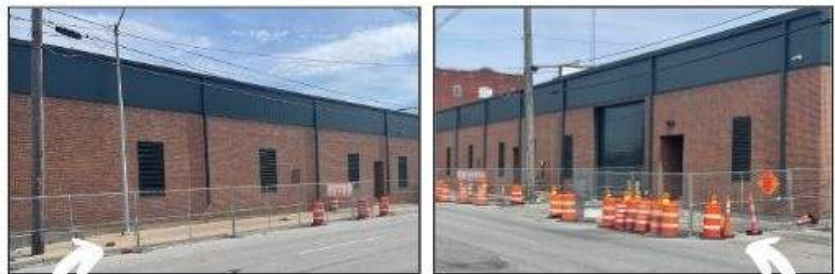
The work-in-progress, taken in April 2025.
